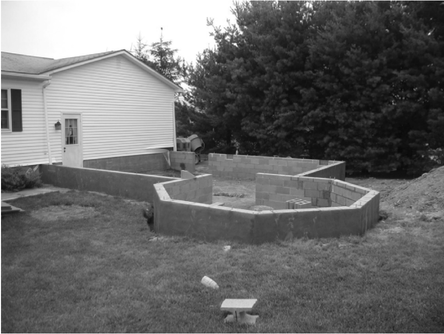
Figure 11.2. The foundation footprint of the addition for the observatory.
