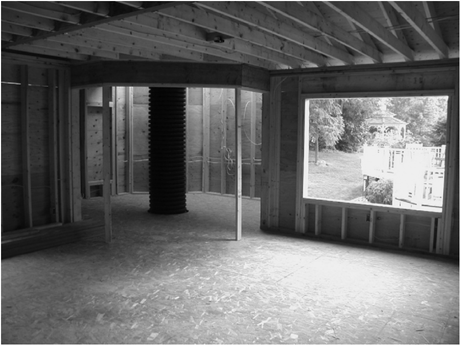
Figure 11.7. The interior of the new addition.
