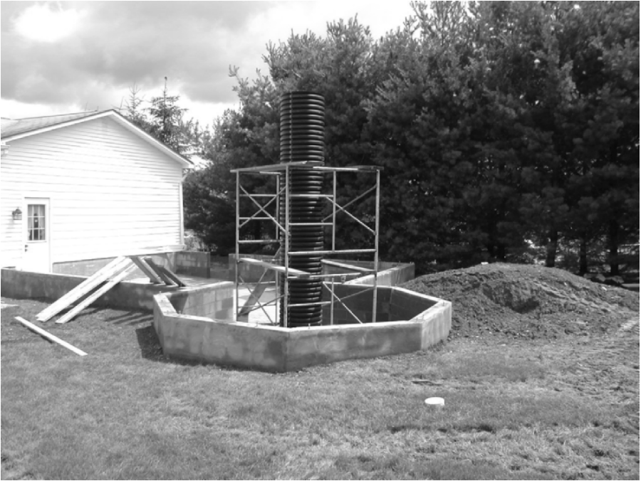
Figure 11.5. The pier tube prior to insertion of concrete.
