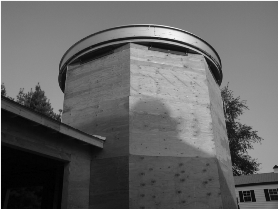
Figure 11.8. The dome skirt will allow the dome to easily spin.
