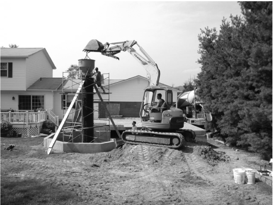
Figure 11.6. The back-hoe delivers concrete to pier by way of hopper.
